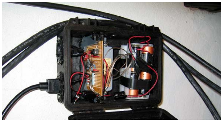
View of J4 Popo microphone deployed inside hut at Popocatepetl using a temporary C-cell internal battery supply (right side). Note the grey electret condenser element box (middle behind the circuit board) and the two cables extending from the AC plugs (left).
